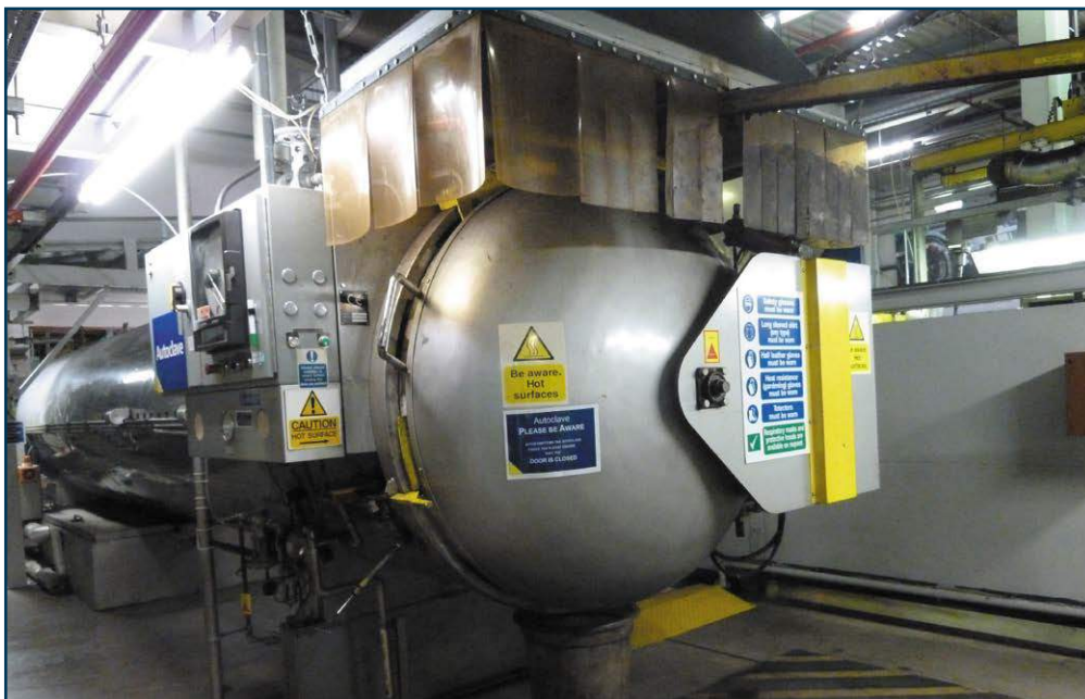
Figure 10 Autoclave with quick-opening door
